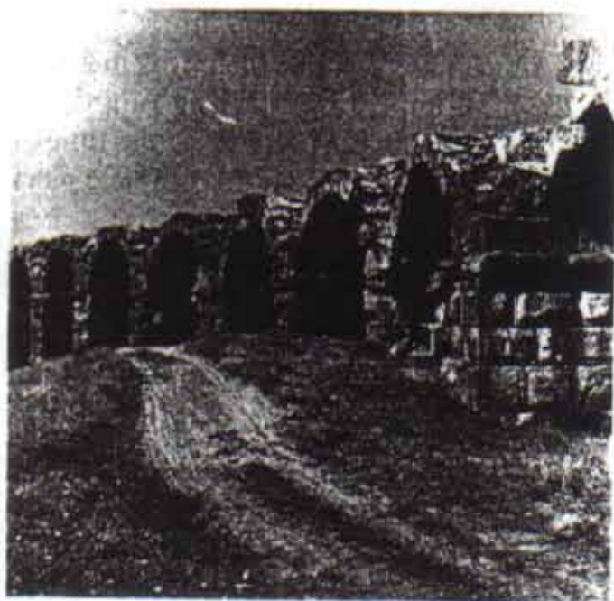
PLATE 124. Aqueduct. Arches a20-a27 (Ballance).
