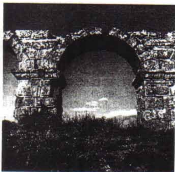
PLATE 129. Aqueduct. Piers p5 and p6 with cornice type C1 (Ballance).
