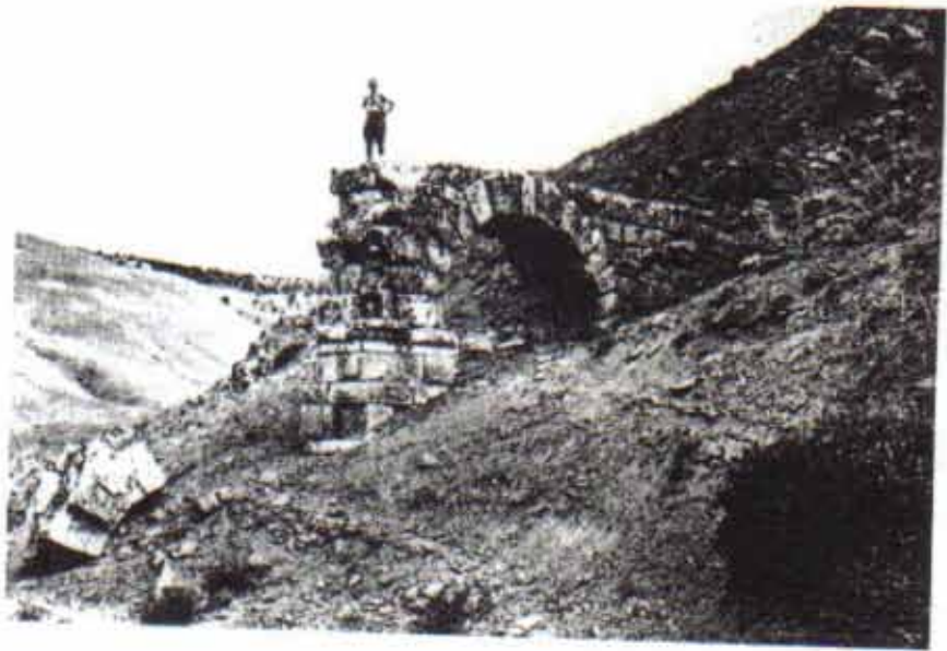
PLATE 122. Aqueduct, Bridge P2, fifth pier and arch from the north (Kelsey archive 7, 1358).
