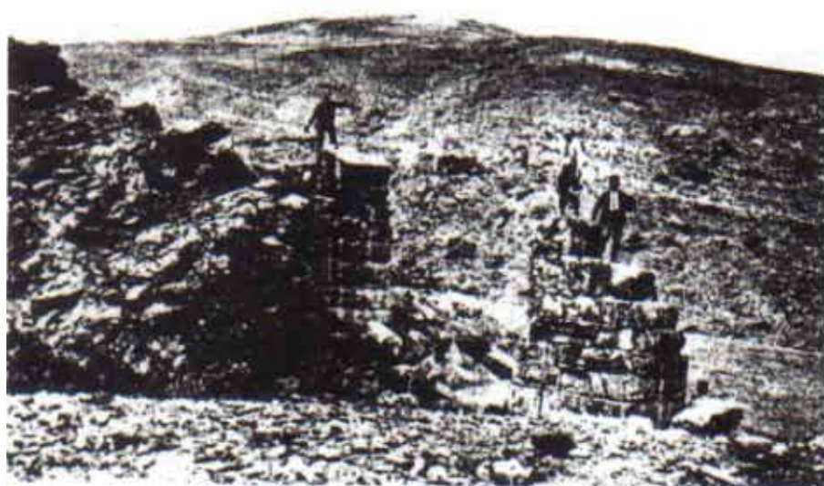
PLATE 121. Aqueduct. Bridge P2, abutment and first pier from the north (Kelsey archive 7. 1357).
