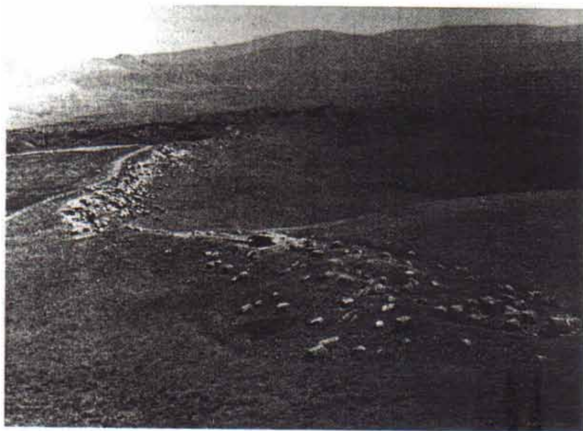
PLATE 127. Aqueduct. The siphon from the city wall (Ballance).
