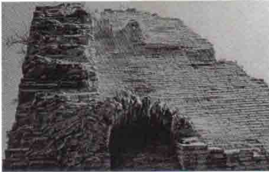
Fig. 15. Brick part of south tower, remains of vaults on which stairs led to the top.
