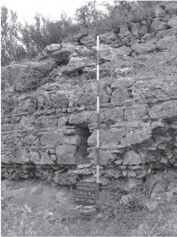
Fig. 9. Outlet 14 for rain water in the older line in section XI.
