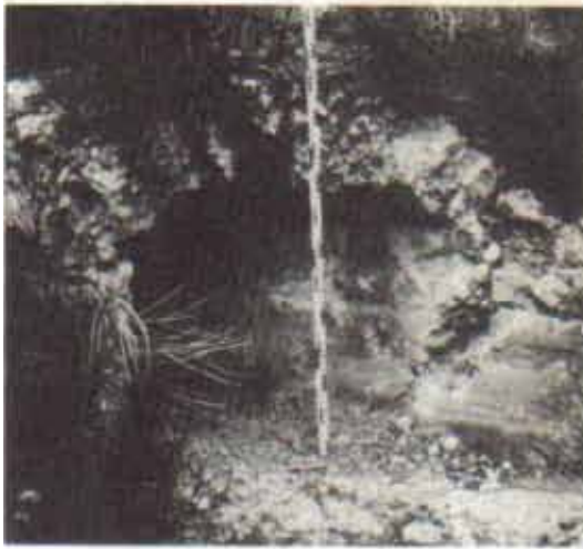
Fig.15 Channel of cast Roman concrete -Aix-en-Provence-
