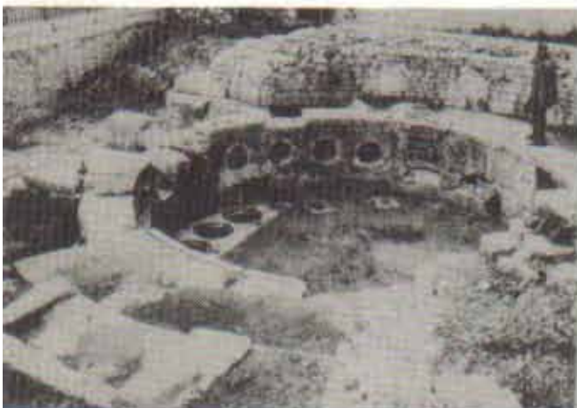
Fig. 19 Distribution structure - Nimes -
