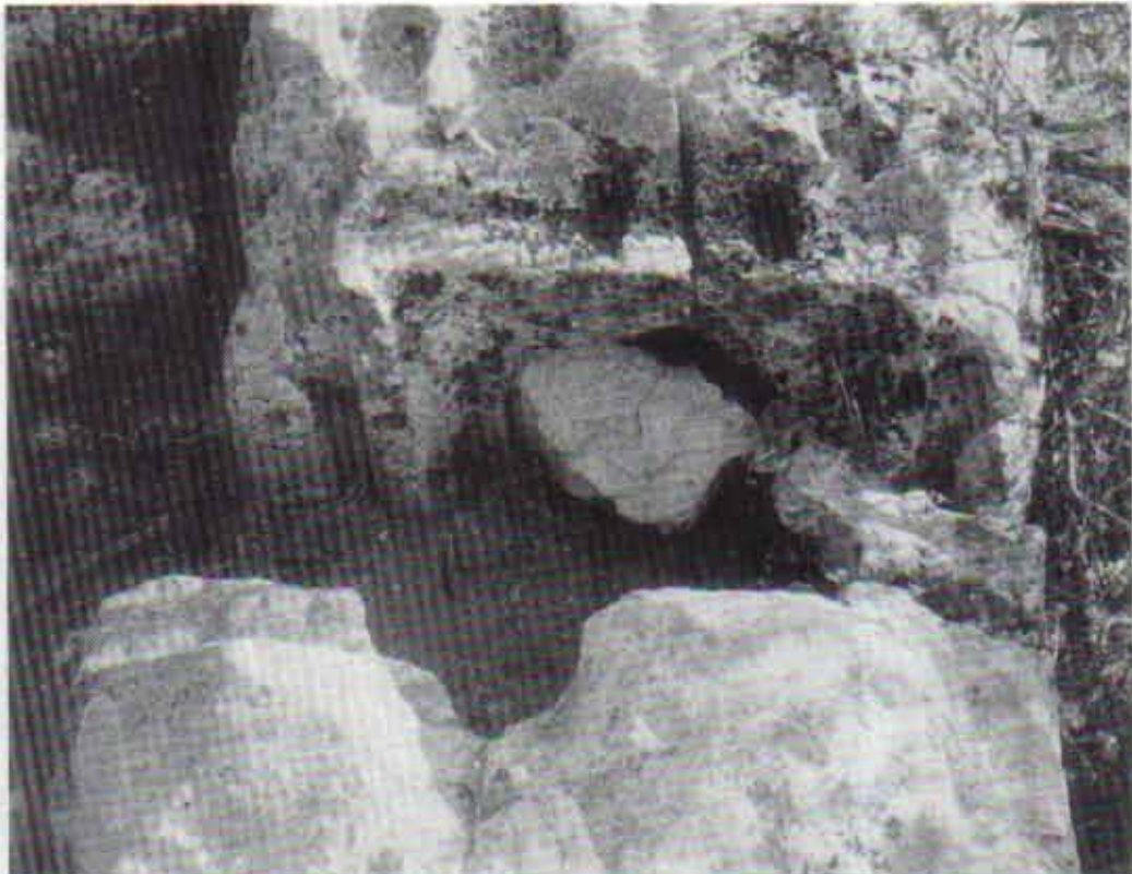
2 b. Patara: recess for metal sluice (?) at southern end of sloping section of stone pipeline (Fahlbusch)
