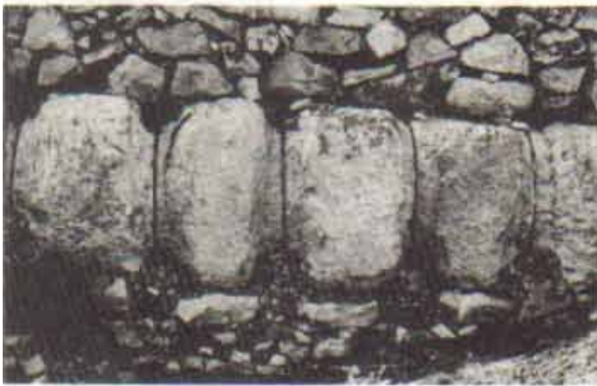
Fig. 17 Pressure pipe-line near Bethlehem
