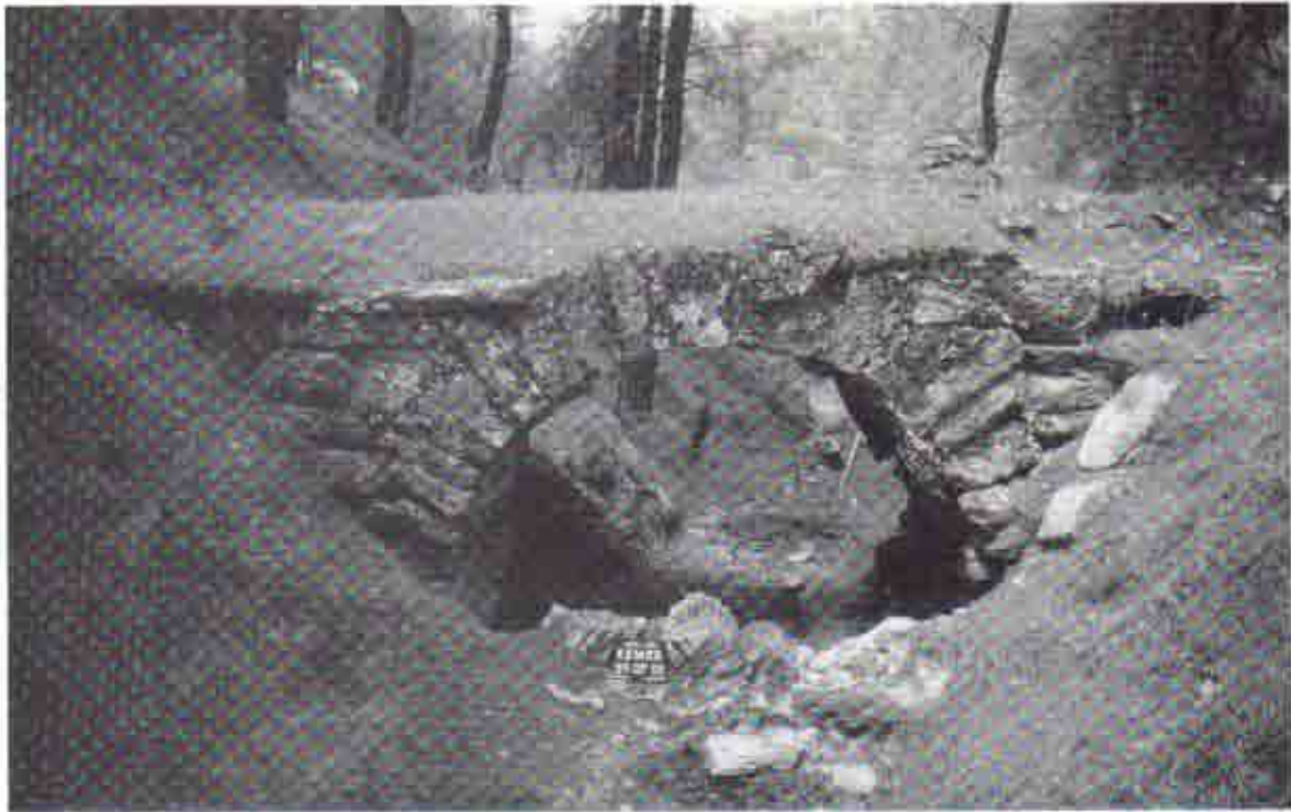
Fig. 9 Small bridge on the Yörükyurdu Deresi. View to southeast. Dia Troia 45971.
