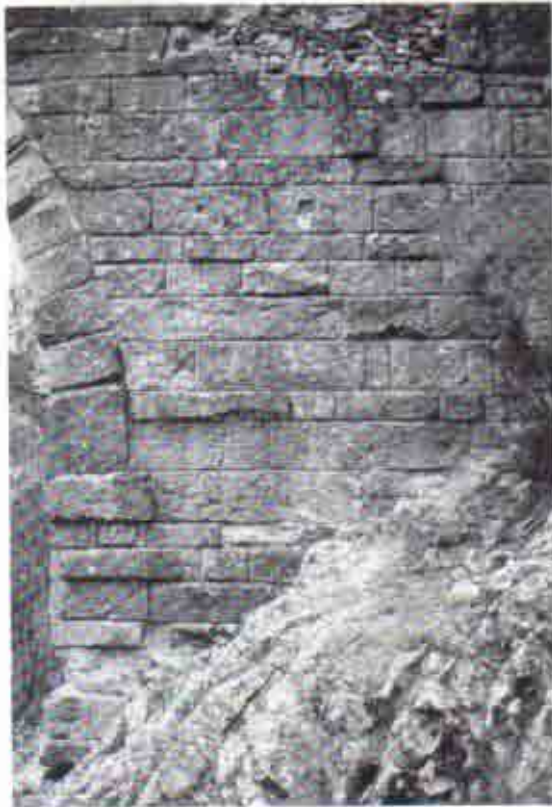
Fig. 15 Detail of the northwest abutment, northeast face.
