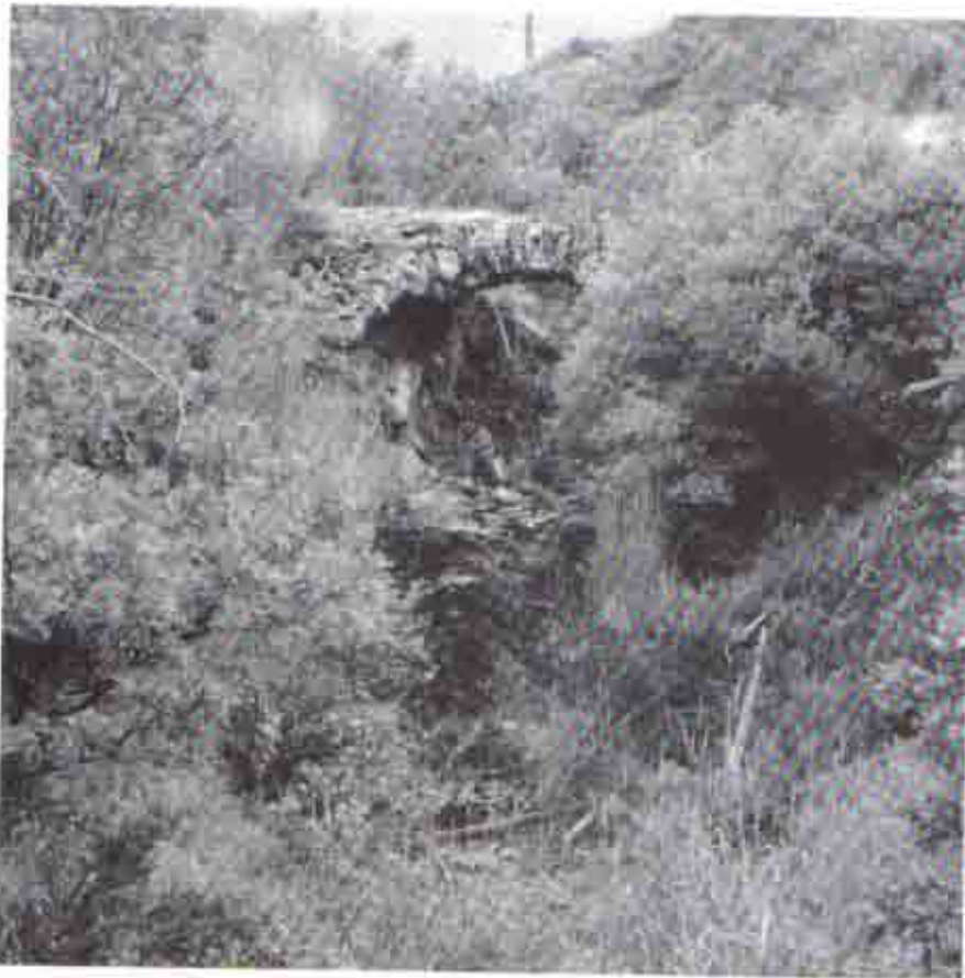
Fig. 5 Small bridge on the Suçıklı Deresi. View to southwest. Dia Troia 45968.
