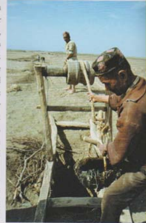
Vertical Shaft of Karez (ground working)
