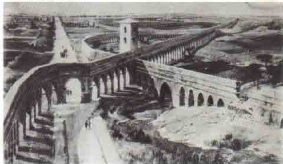
Fig. 10. Intersection of the course of five aqueducts near Rome (painting by Zeno Diemer, Deutsches Museum, München)
