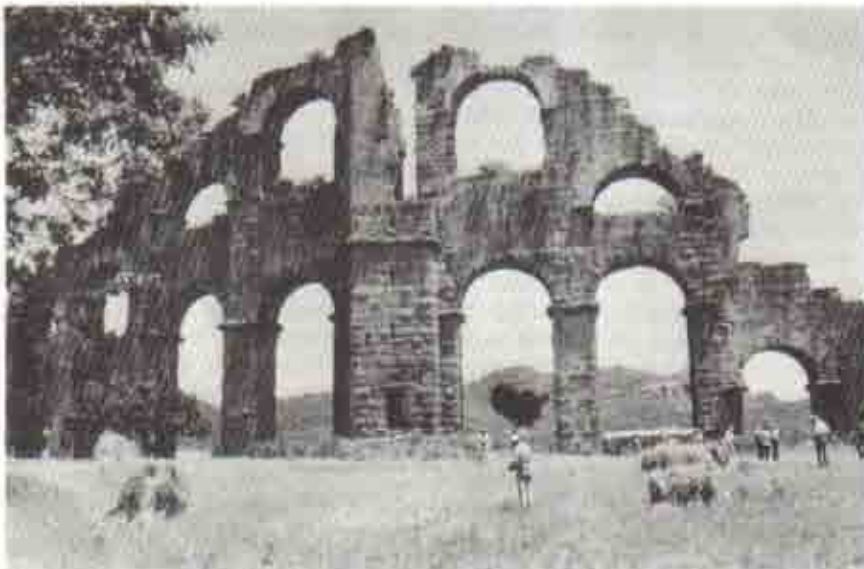
Fig.6. Tower in the pressure conduit near Aspendos/Turkey
