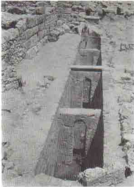
Fig.8. Cisterns at Ampurias/Spain (Photo: Lamprecht 1984)
