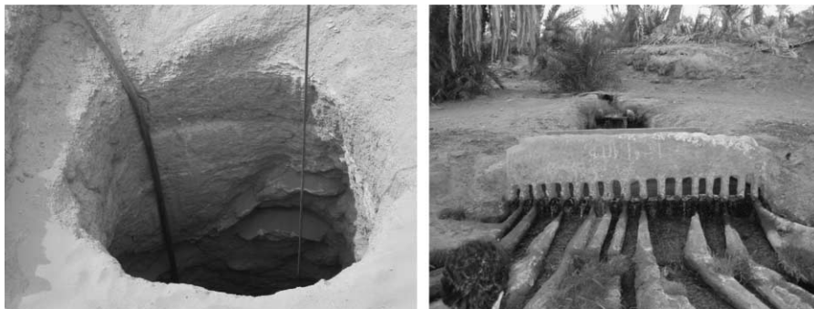
Figure 1 A foggara at Adrar, Algeria: (left) shaft; (right) distribution and metering weir at the foggara outlet
