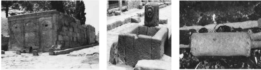
Figure 9 Elements of water supply system at Pompeii: (left) castellum divisorium at Porta Vesuvii housed in the large brick building; (middle) public fountain; and (right) lead pipe with enlarged section of junction box
