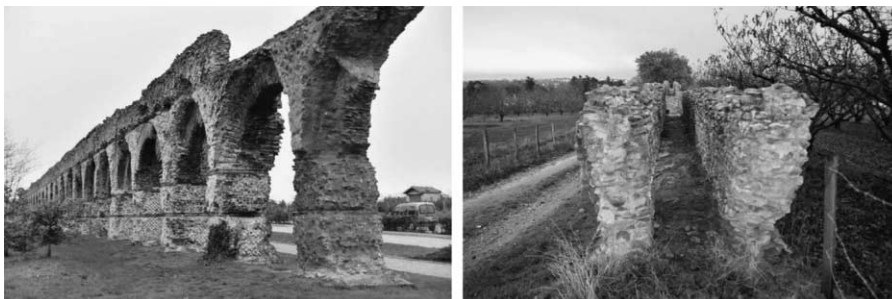
Figure 6 Aqueduct of the River Gier near Chaponost, France
